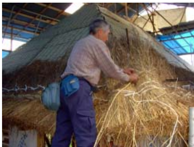
Figure 3 Master M. thatched from the eave to the top in the traditional manner almost all by himself.
