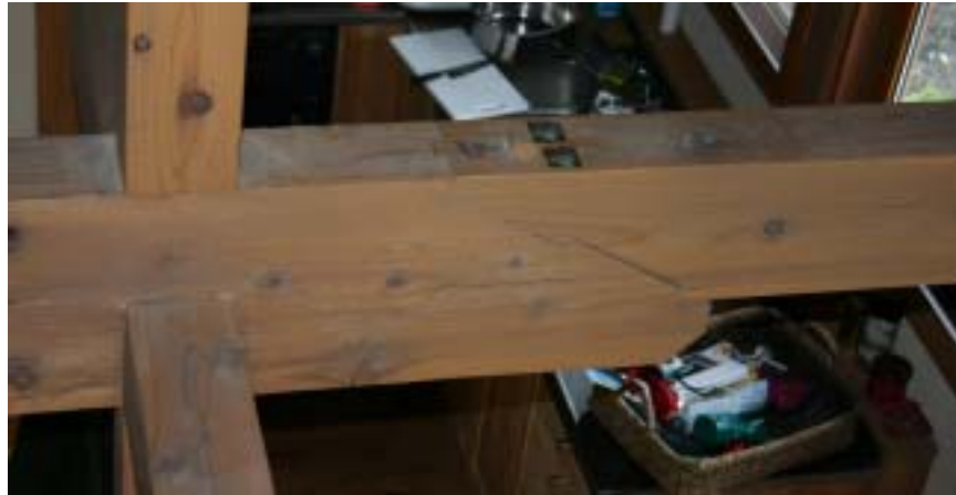
Figure 5 The simply screwed breakage of the suspended joint of beams.
