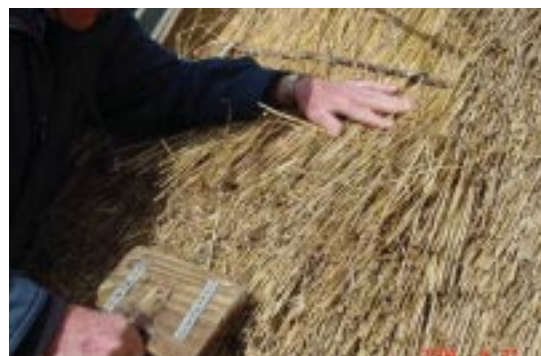
Trimming the straw with a shears Co. Galway
