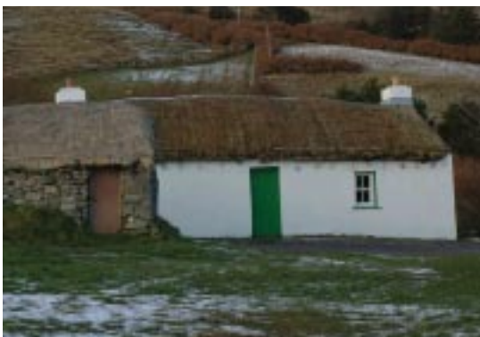
Roped thatch buildings Co. Donegal
