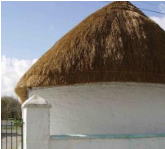
Scollop thatch- ing with straw on hip-roof house Co. Offaly
