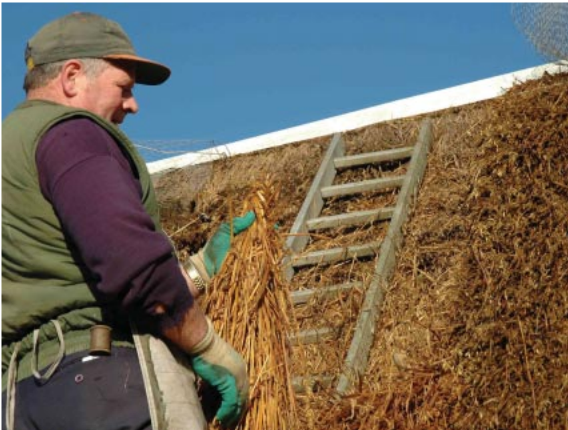
Nick Furlong preparing the 'dull' for thrusting into the roof
