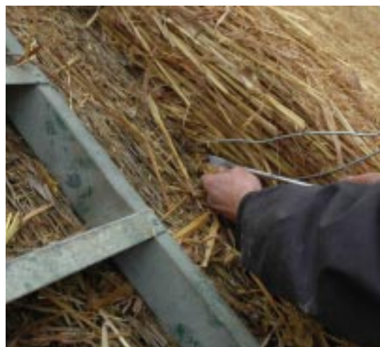
Left: John Brereton thrusting the straw into the roof Co. Kildare
