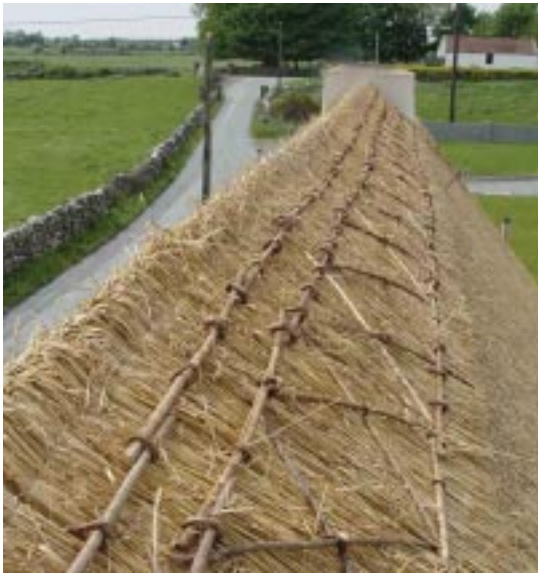
Finished ridge with bobbins and stretchers Co. Galway
