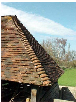
Petersfield brick drying shed
