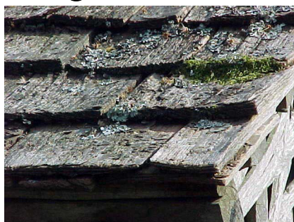
Detail of the shingled roof of the beehive shelter in Bayleaf garden
